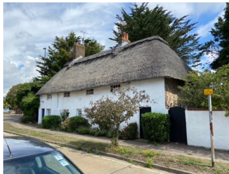
Fig 16: Thatch, render, brick and flint concealing earlier timber frame at Connaught Avenue
