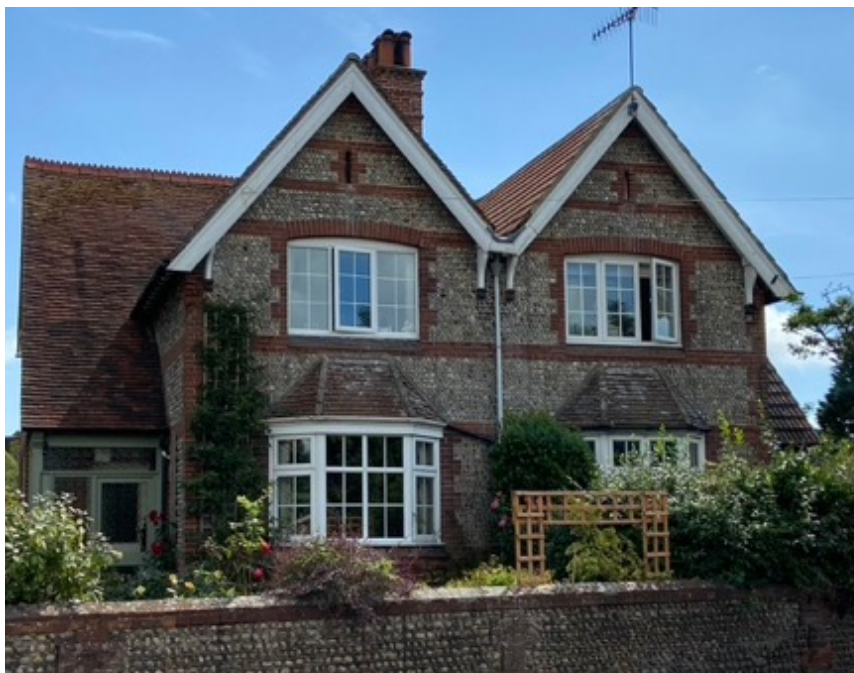
Fig 30: Modern uPVC windows to unlisted historic buildings
