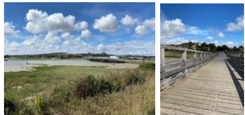
Fig 7: Old Shoreham Toll Bridge
