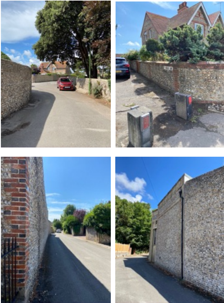
Fig 19: Historic flint walls
