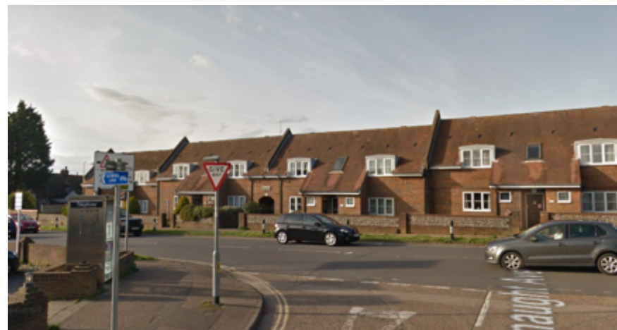
Fig 31: Modern development on Upper Shoreham Road; poor quality street furniture
