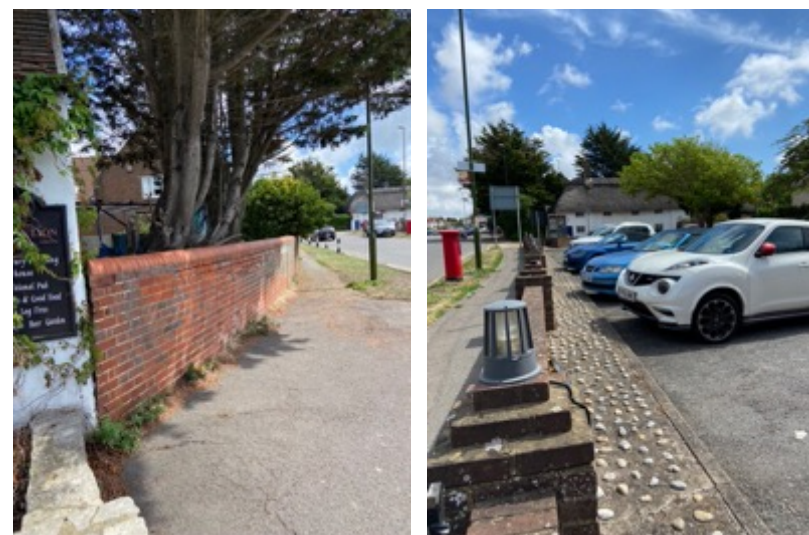
Fig 34: Modern inappropriate brick wall and boundary treatments
