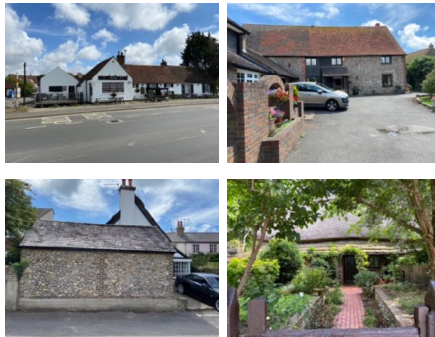
Fig 18: Various roof materials: thatch, clay tiles, slate, Horsham slab
